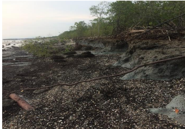
Figure 7: Erosion effect at coordinate 1;41;15.152200, 103;5;44.929999
