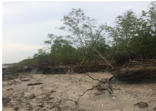
Figure 8: Erosion effect at coordinate 1;41;13.886499, 103;5;46.335399
