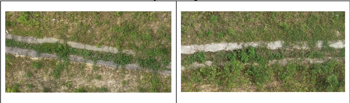
Figure 9. The vegetation growth on slope and the silt in drainage at Jalan Bangi
