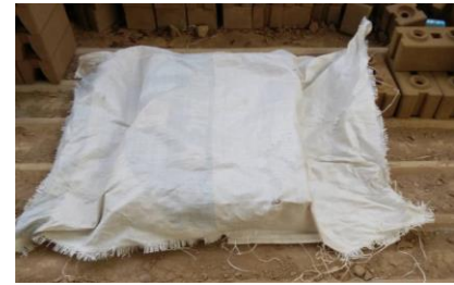
Figure 8. Covering the ICB with tarpaulin (Curing C).
