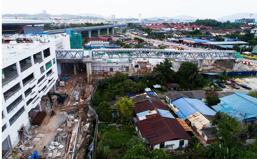
Figure 1: MRT station being built alongside the remaining village of Kampong Bukit Dukung at Jalan Cheras, Kajang in 2017.
